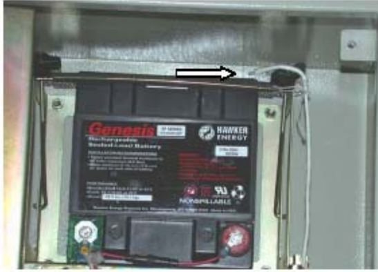
Figure 6: Location of top temperature sensor inside of the test sample
